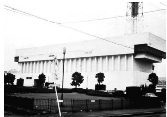
Garbage incinerator facility
